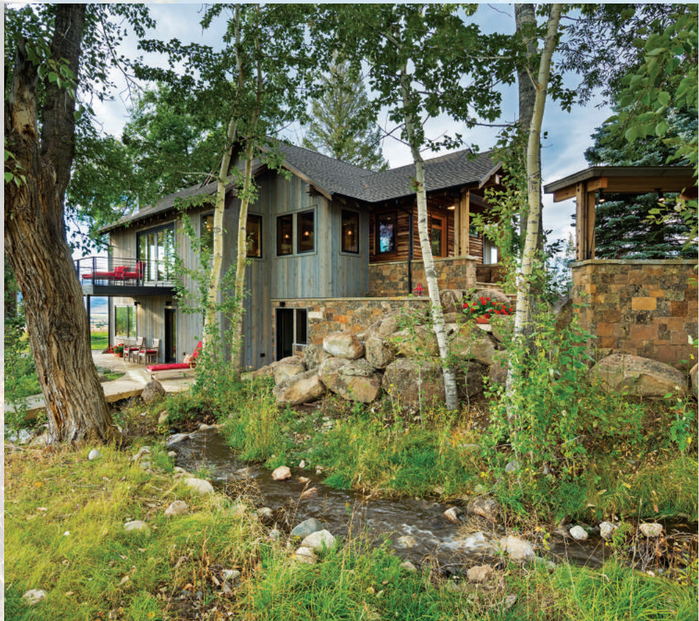
ABOVE: The homeowners wanted the outdoors to feel like a part of their home environment. A quick trip outside to cook dinner on the grill helps achieve this effect. RIGHT: The design team worked together to remove the old farmhouse and modernize the foundation, which had previously flooded and was sheltering "a pretty hardy mouse population," according to Rudolph. The home's footprint remained essentially the same even while the flow and functionality were substantially improved.
